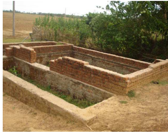
AWC building at Sasanpada, GP-Chikana (PS Binjharpur)
