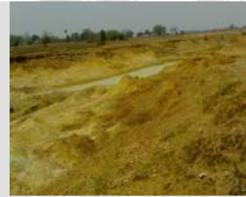
Failure zones of SMC 7950 to 8720M
