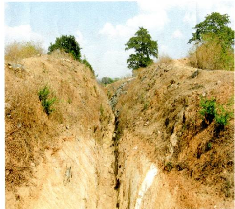
Incomplete branch canal system
