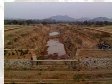
Left Main Canal (head reach) of Lower Indra Irrigation Project
