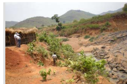
Abandoned site of the spillway of Telengiri Irrigation Project
