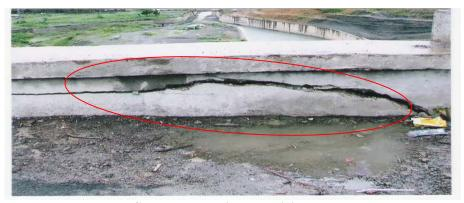
Crack developed in the retaining wall
