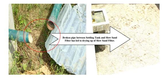
Broken pipe between Settling Tank and Slow Sand Filter
