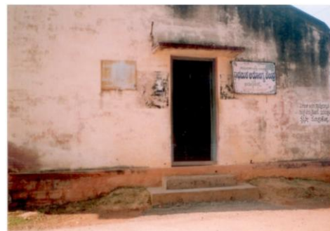
PHC, Araluguppe (Tumkur District) running without proper building (March 2009)
