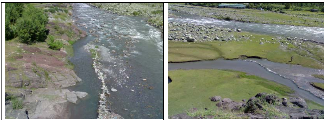
Regulatory System of Chaktroo Khul not installed
