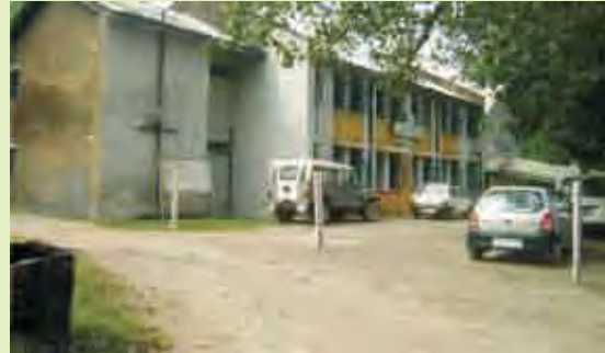
Primary Health Centre Bhota without boundary wall
