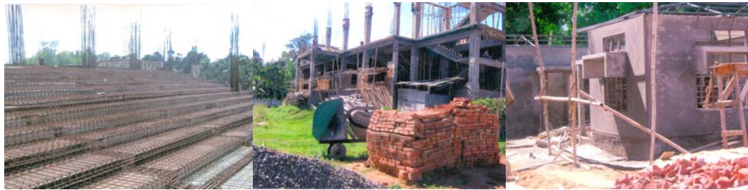
(Gallery, Front Elevation and Caretaker's Quarter of Joi Sing Doloi Auditorium Complex)
