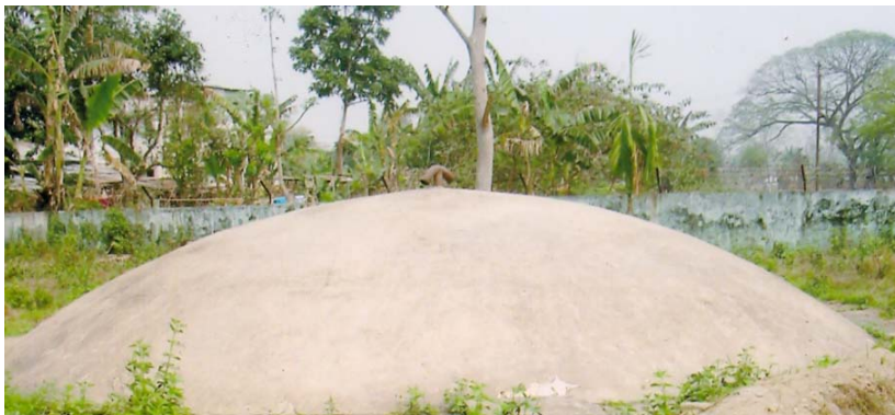
Clear water sump of Dergaon TWSS
