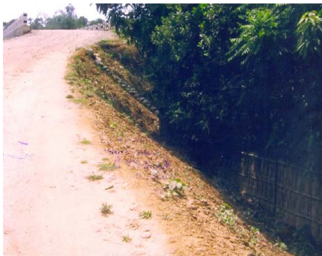
RCC Bridge No. 15/1 on Silchar-Kumbhirgram Road
