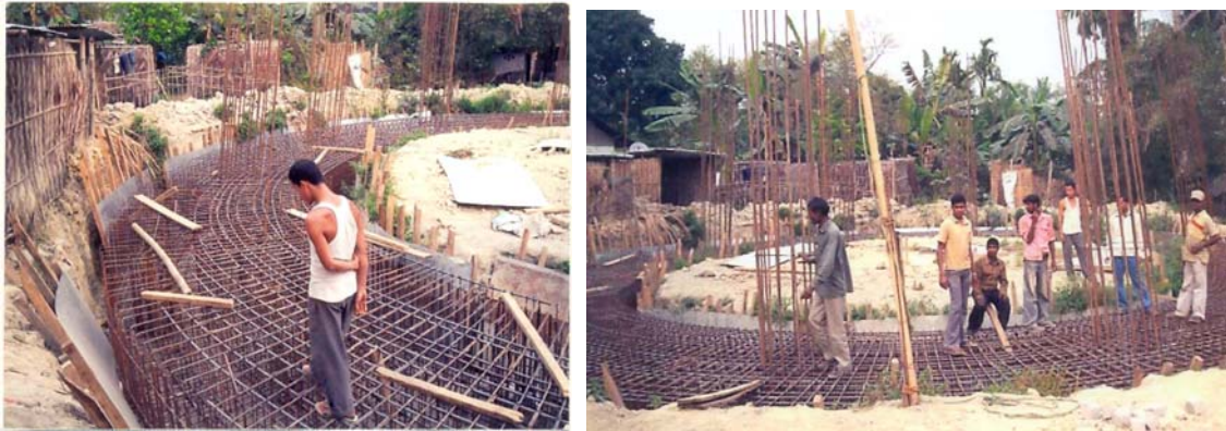
Overhead Reservoir No-2 of Golaghat WSS
