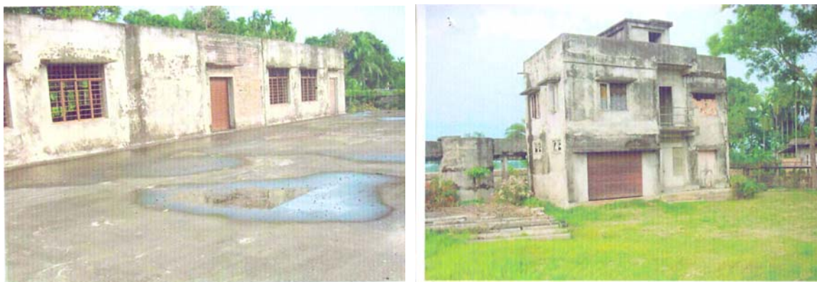
Clear water sump and, Chemical house of Gauripur WSS
