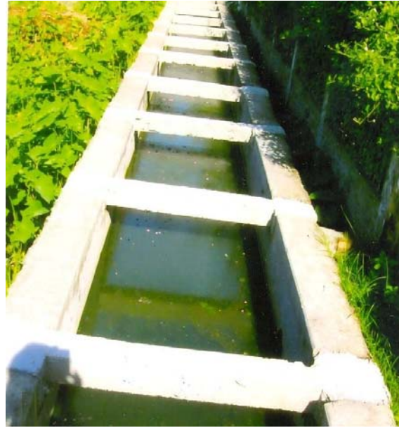
Drain No-7/Along Chandmari Bye Lane No-2
