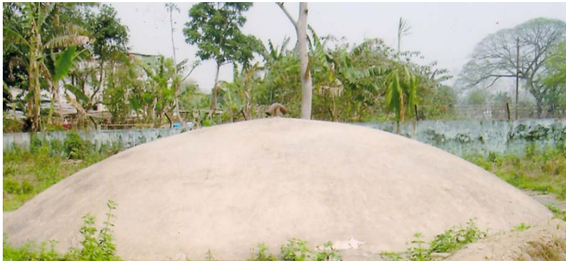
Clear water sump of Dergaon TWSS
