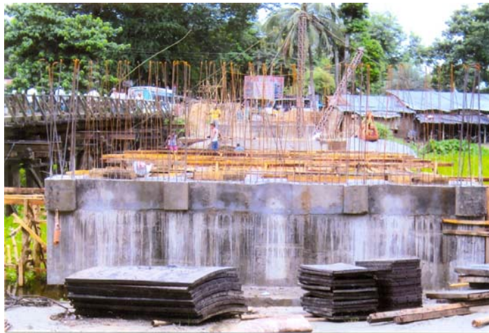
RCC bridge No-1/1 over river Shantijan
