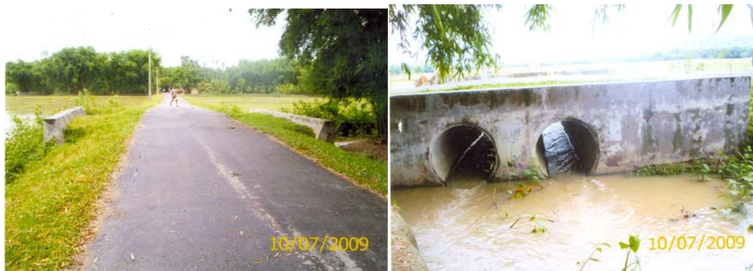
Construction of RCC bridge No-10/5 on Gar Ali Border Road
