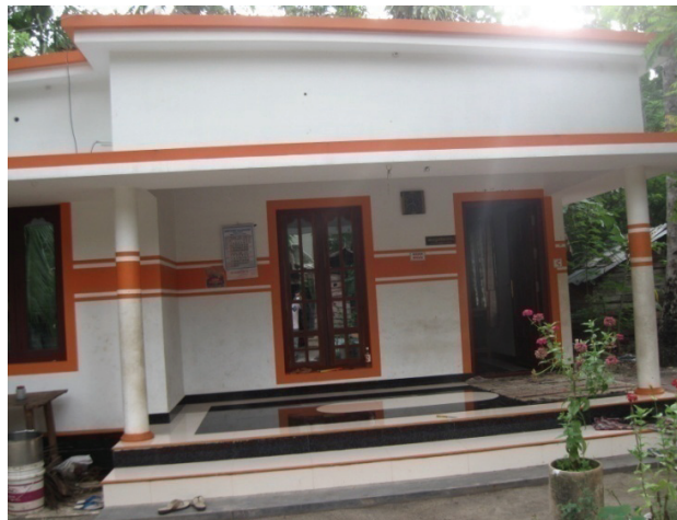
IAY house costing more than ₹ 4 lakh
