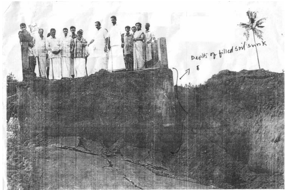
View of sunken approach road at Kannadichal
