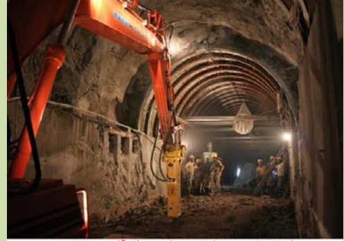
Tunnel T1/P1 Rectification work in progress (Photo on 21/09/2010)
