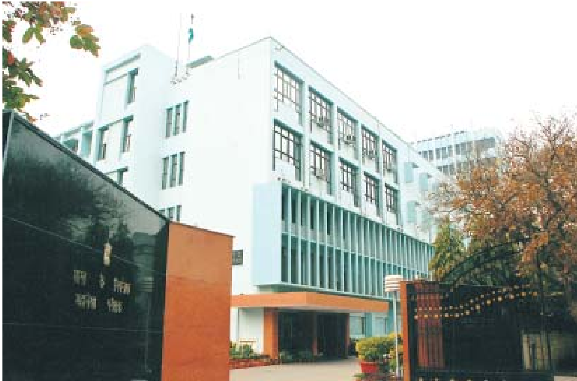
The present Headquarters of the office Comptroller and Auditor General of India at New Delhi.
