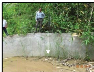
Blocked sluice due to siltation
