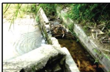
Seepage and blockage of lined channel
