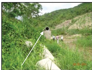
Broken hume pipe channel
