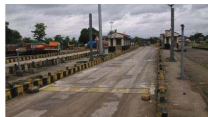
Non-functional weighbridges with damaged installations
