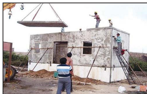
(Picture showing erection of precast panels for CCP/COP)
