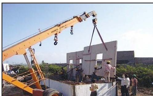
(Picture showing erection of precast panels for CCP/COP)
