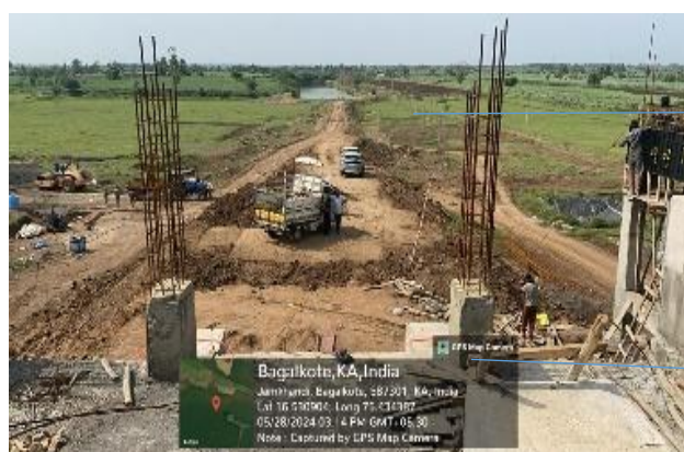
Image 3: Change in site of Jack well from location A (left unutilized) to Location B. And work in progress of Jack well (as per new design).
