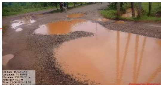
Picture No. 3: Damaged road at Kittur IA
