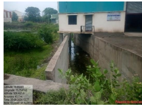
Picture No 15 & 16: Plot no. 54 land measuring 1000 sq. meters in Aliyabad Block-II- Construction of buildings encroaching storm water drain.
