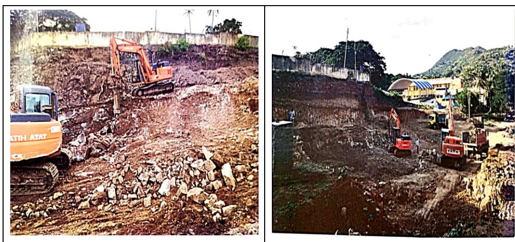
Picture 31 and 32: Excavation using mechanical means in Chamarajanagara
