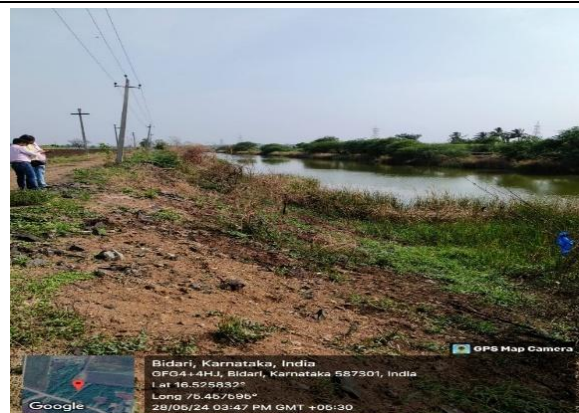
Image 2: Excavated Intake well (as per old and left unutilised due to shift in location of the Jack well.
