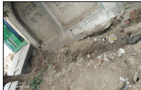
Photographs 6 and 7: Dumping of waste in drains and choked drains in Bawana IA, as observed during joint physical verification in December 2019
