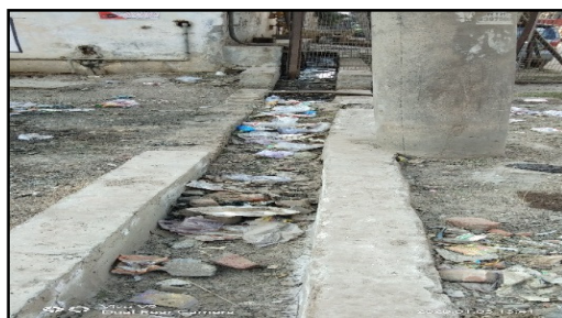
Photographs 4 and 5: Choked drains and overflowing drains in Narela IA, as observed during joint physical verification in January 2020
