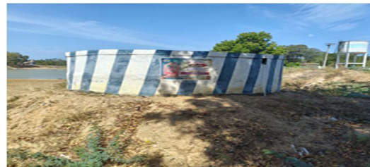
Exhibit 2.2: Open well at Thinaikulam VP not used
