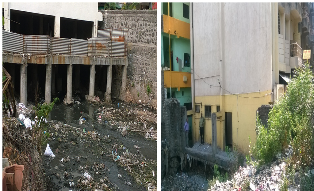
Picture 5 and 6: Unauthorised constructions
