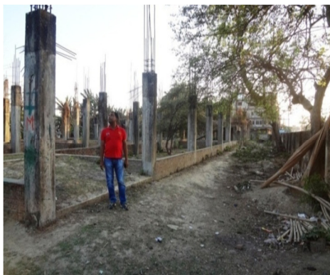
Four storey RCC building of General Nursing Midwifery (GNM) School-cum-Hostel at Nagaon (30.06.2016)
